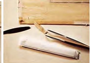
Detachment and removal of adhesive residues.
